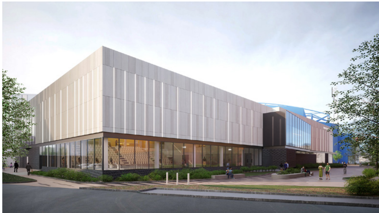
VIEW FROM FRIARS BRIDGE RD TOWARDS SOUTH - WEST
