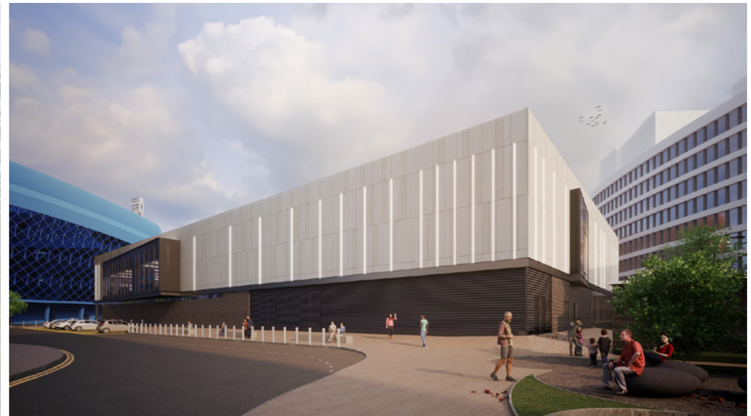
VIEW FROM PRINCES ST TOWARDS NORTH - WEST
